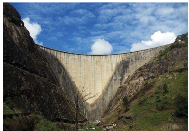
Fig. 2. Idukki Arch Dam – Downstream side
